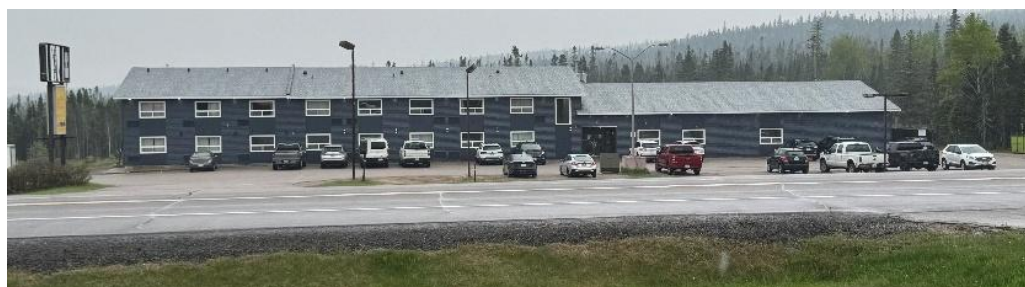
South Side Complex
