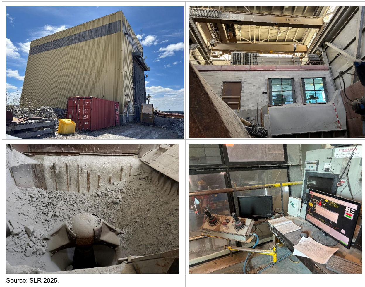
Figure 18-6: Existing Crusher Building
