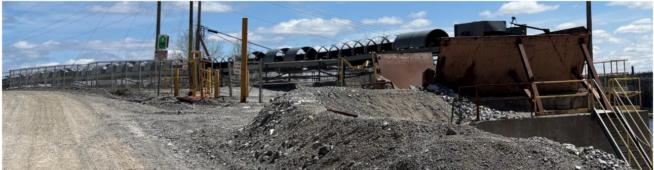
Figure 18-10: Conveyor #19 Discharge to #3 Transfer Station
