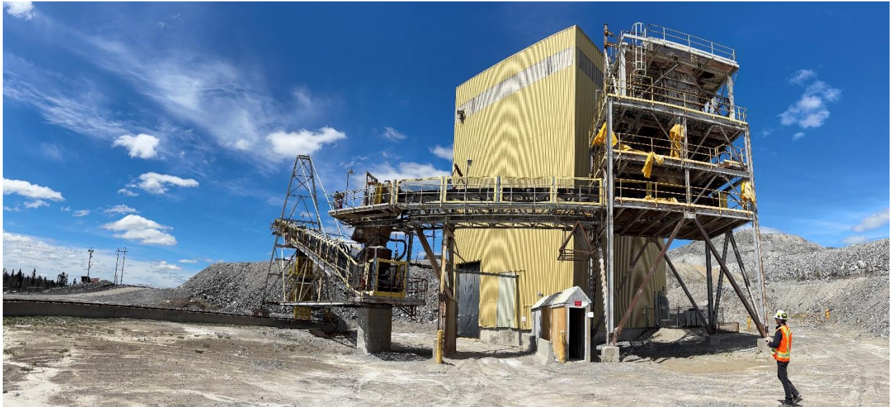
Figure 18-8: Screen Building and Stacker Conveyor
